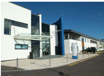
Crosshouse Maternity Hospital, UK
