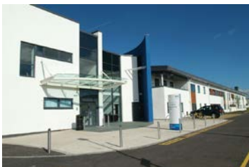
Crosshouse Maternity Hospital, UK
